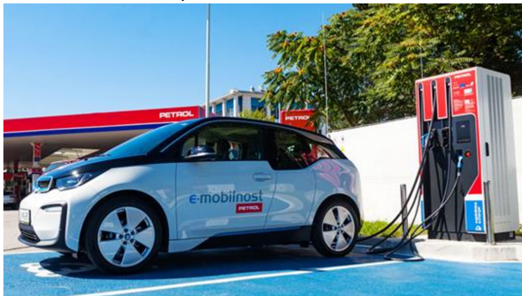
Picture 5: Petrol Fast chargers (DC 50 kW/AC 43 kW)
