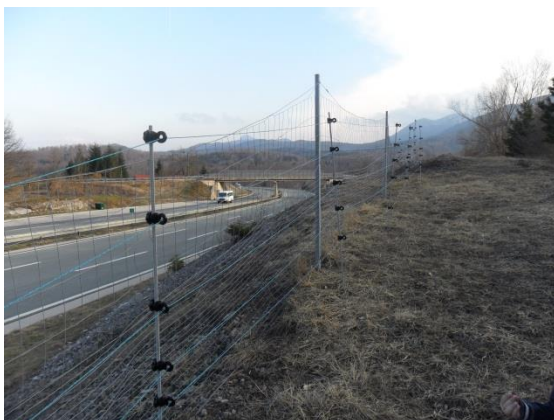
Picture 6 Electrical fence along the highwa
