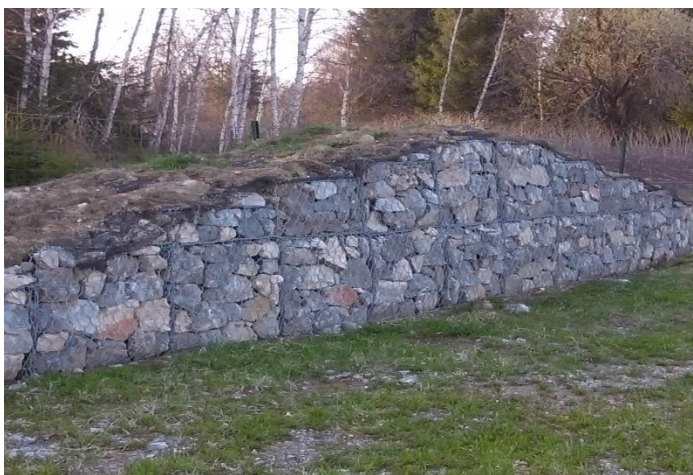
Picture 8 A ramp to exit the animals from the highway
