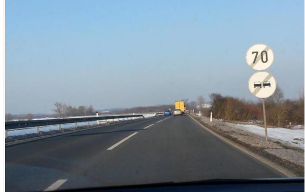
Picture 9. Instead of traffic sign end of speed limit sign "60" there is installed traffic sign end of speed limit "70"
