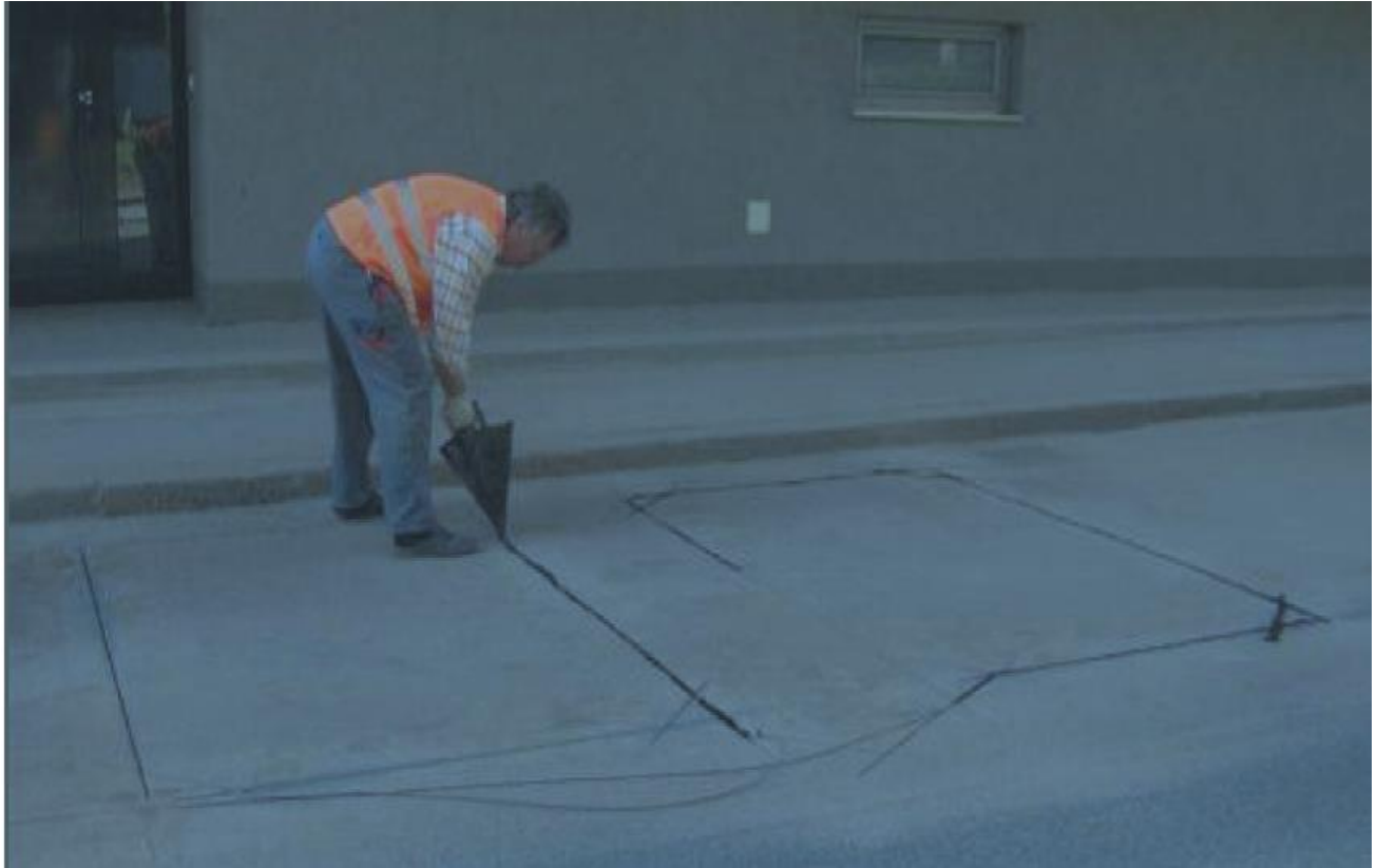
Figure 5: Inductive loop in the road.
