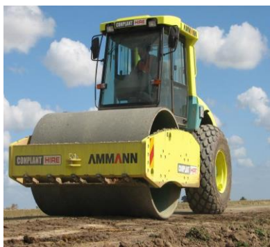
Picture 9: Roller during the work
