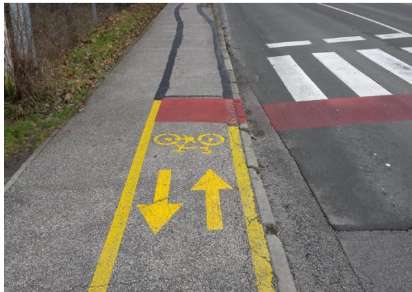
Picture 2. Two-way bicycle path and vertical transition
