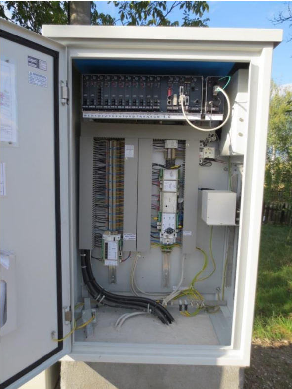
Figure 7: Traffic light system with inductive loop
